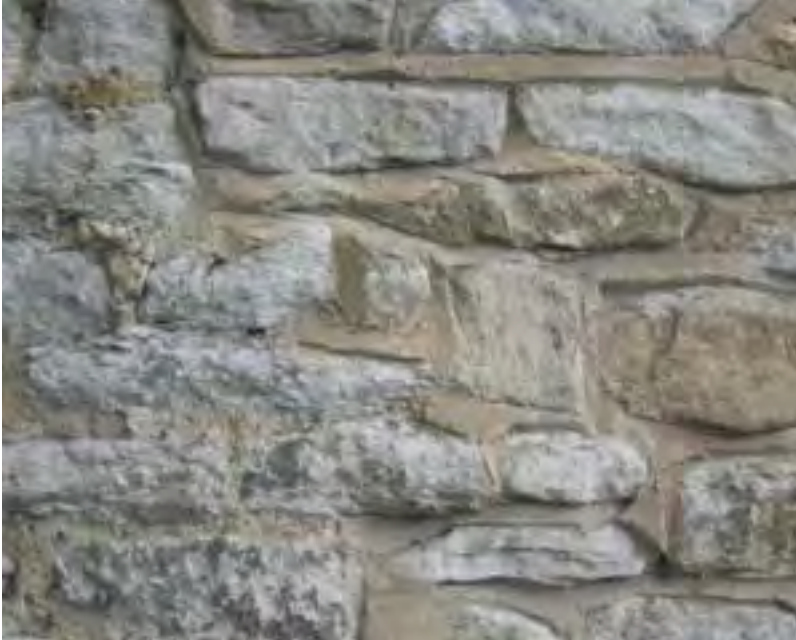
Original lime mortar and cement repointing
