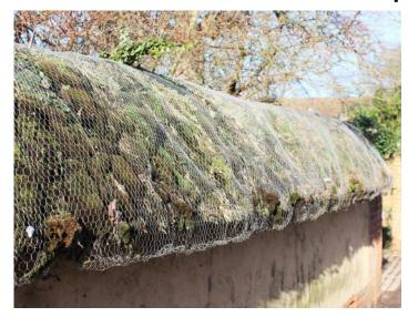
Like all thatch, this roof deteriorates over time and has to be renewed. The state of the thatch at the beginning of tis year can be seen in the first picture.
