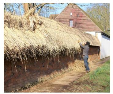
'Cob walls need a good hat and a good pair of boots. The hat keeps the rain out of the cob. Traditionally this was thatch but slate or tiles were also used. The boots were generally a brick, stone or flint plinth, which acted as a damp-proof course.'
